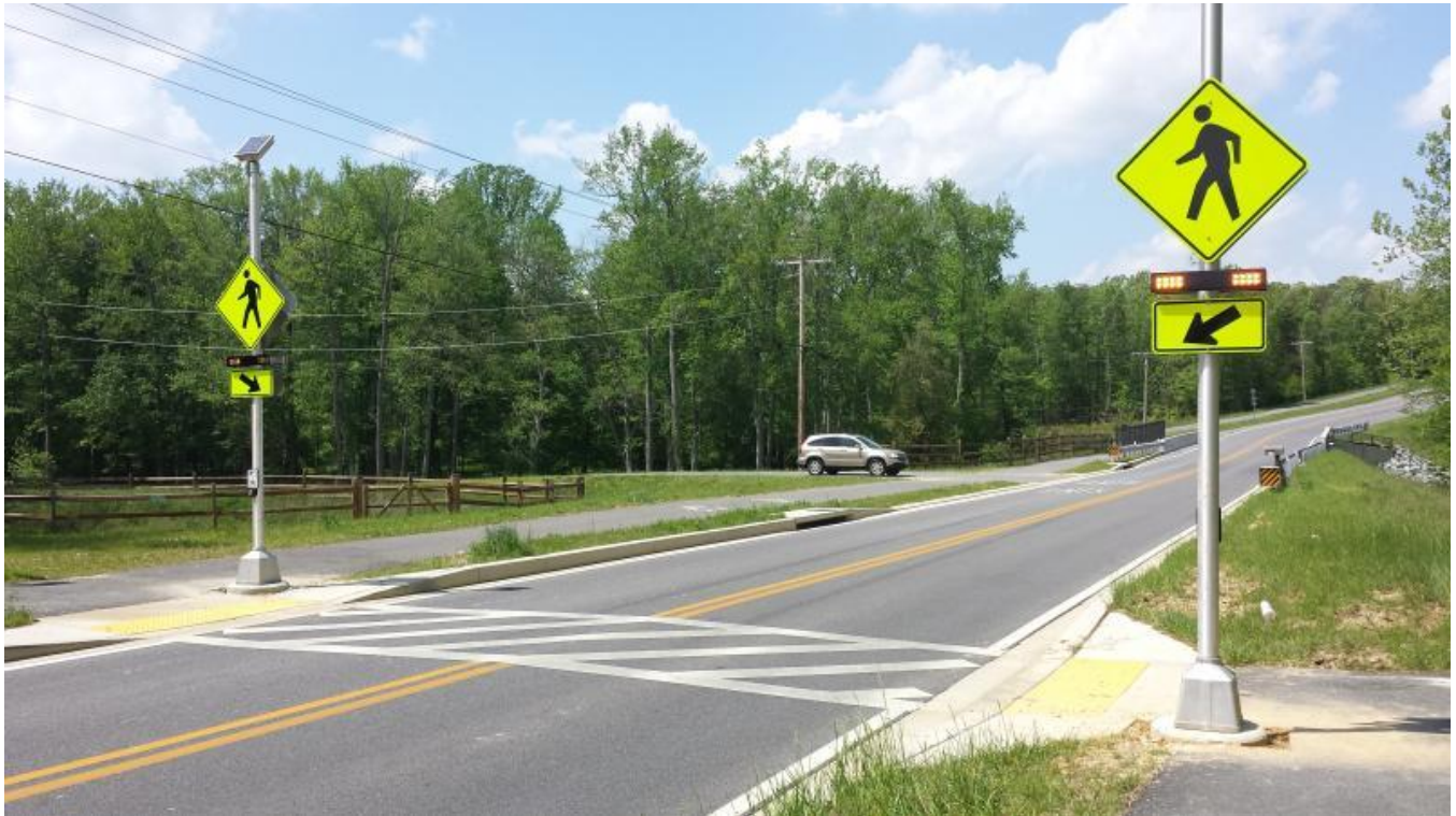
Above: Example of a rectangular rapid flashing beacon (RRFB). Lights flash on the crosswalk signage when a pedestrian hits a button at the bottom of the pole, prompting greater visibility of the crosswalk and increased adherence to laws about vehicles stopping for pedestrians in a crosswalk.
